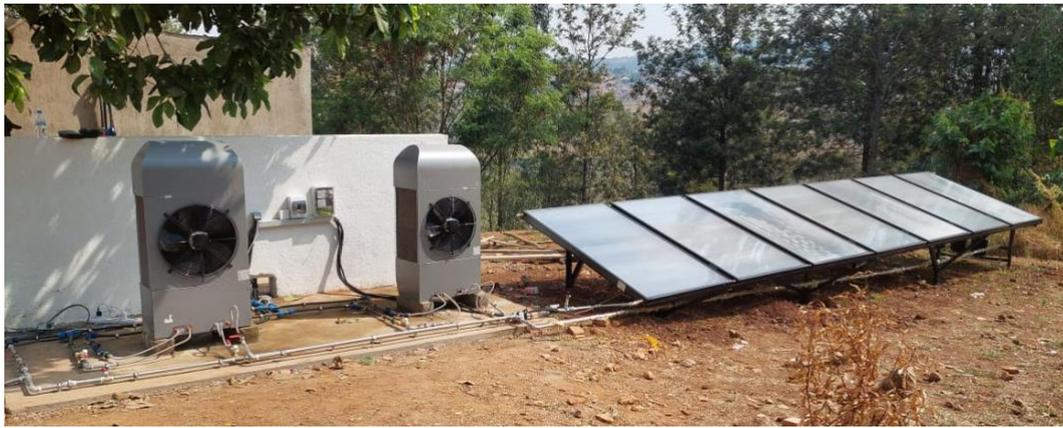
**Figure 6: PURIX 5 kW solar cooling system for a cold storage room installed in Kigali, Rwanda, Source: PURIX.**
